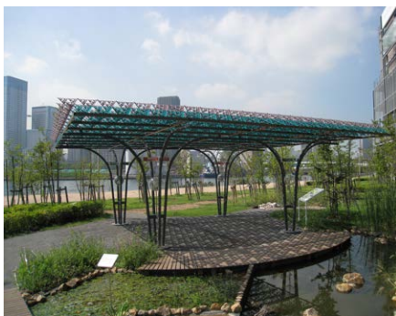
Fractal sunshade material Airyshade developed from the study of the cool shade of trees
